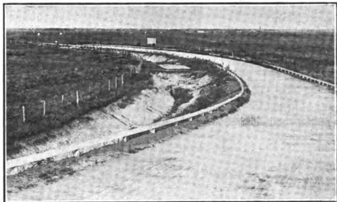
Going toward grand stand, which is about 1 1/4 miles away
